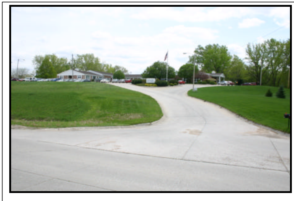
Photo 2 - Louisville Care Center entrance looking southeast.
